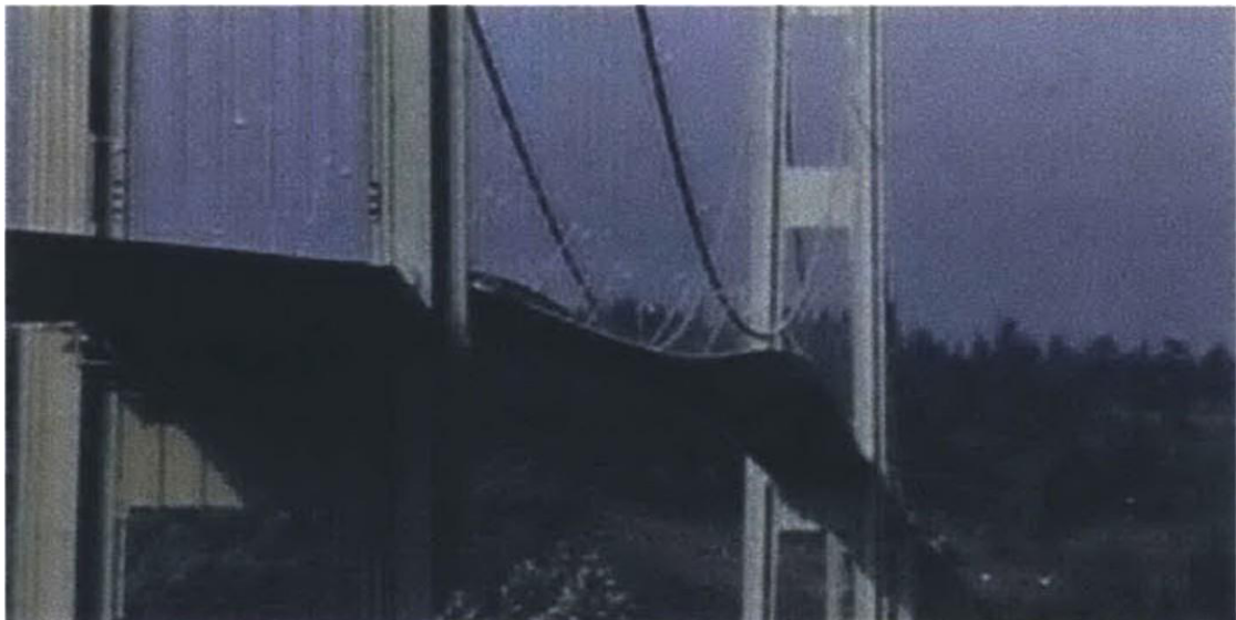
Figure-1. Resonance-Induced Severe Deformation and Eventual Collapse of the Tacoma Narrows Bridge.
